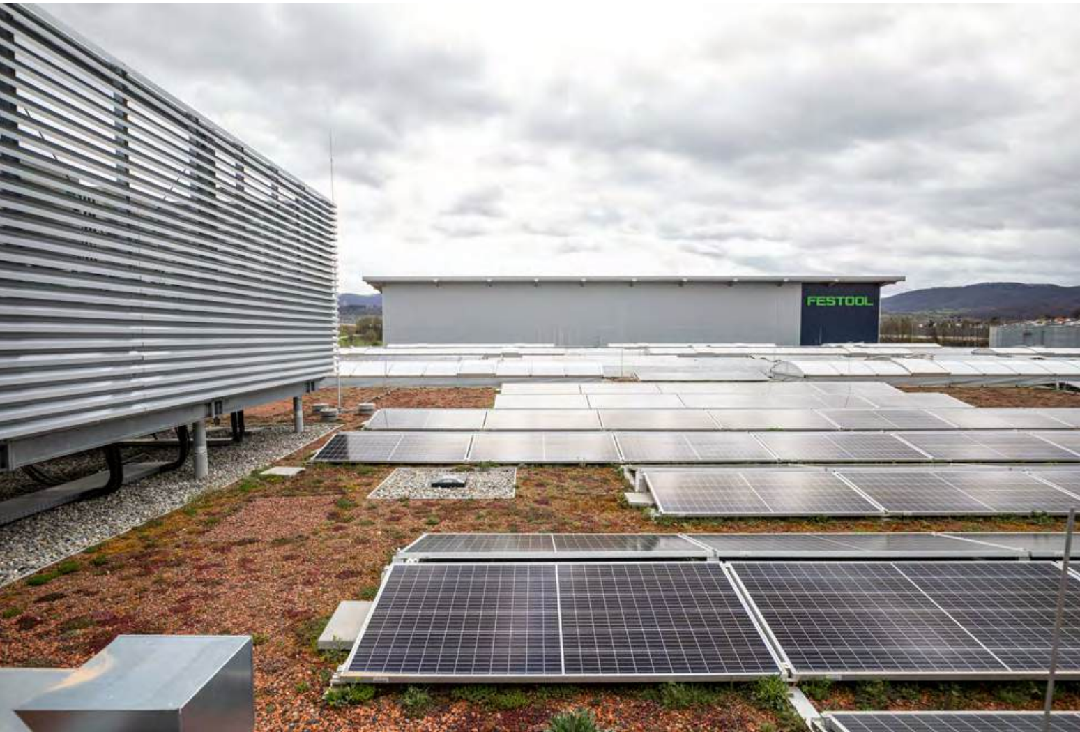
The photovoltaic system on the roof of the assembly hall in Weilheim with a capacity of 600 kWp supplies the entire production site of Weilheim with its own electricity, achieving net zero.
